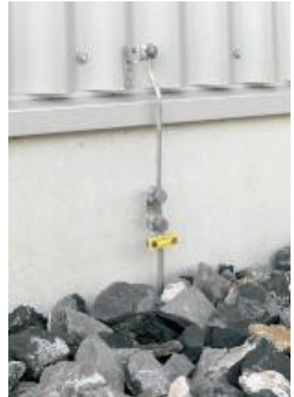
Separation point in an earthing system
