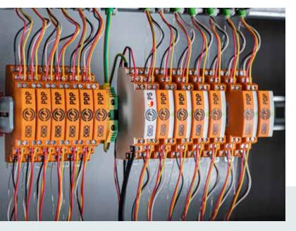
The universal data cable protection devices of the type PDP supplement the OBO portfolio of measurement and control technology protection with a product series with plug-in arresters.
